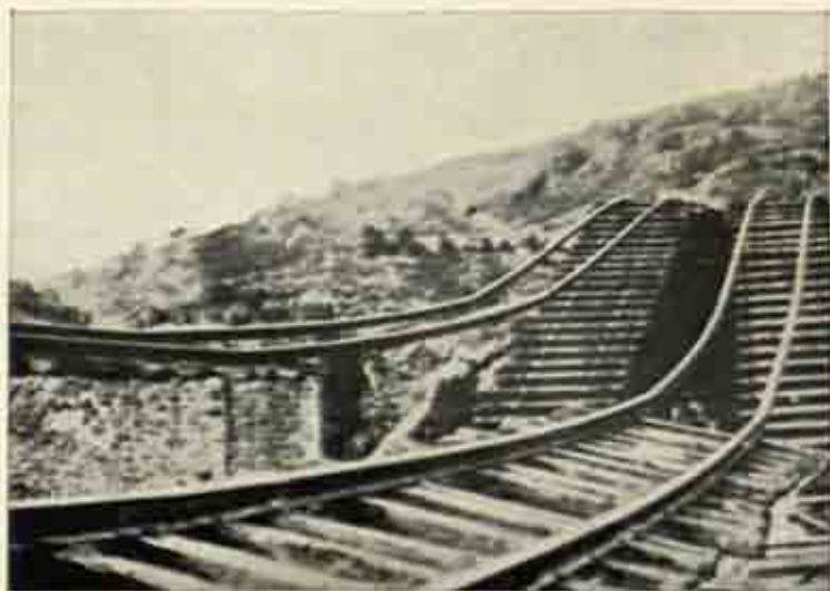
(B) Buckling of railway lines near Tokyo
